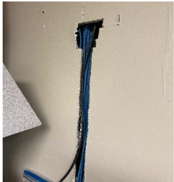
Photograph 4: Exposed wiring
