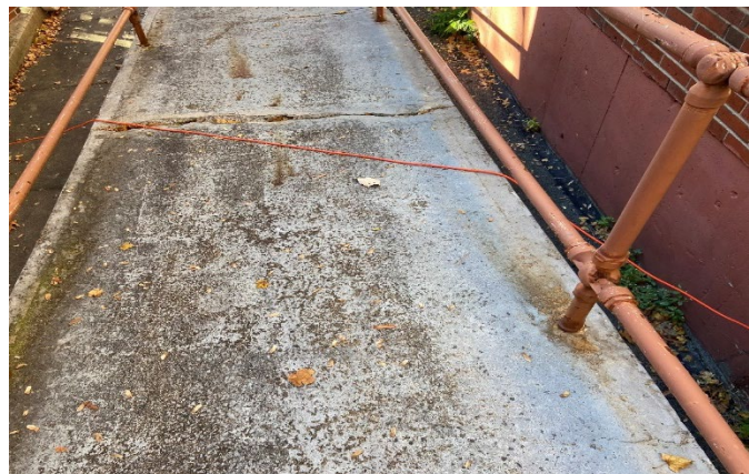
Photograph 8 (left): Unsafe extension cord leaving basement window. Photograph 9 (right): Unsafe extension cord across outside exit ramp.
