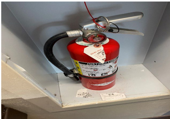
Photograph 5 (left): Fire extinguisher missing monthly inspections tag. Photograph 6 (right): Sprinkler head obstructed by storage boxes.
