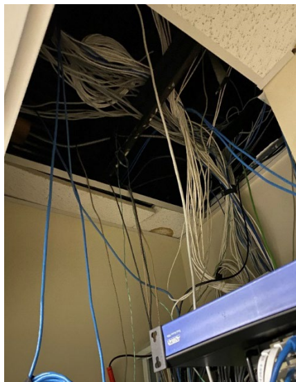
Photograph 1 (left): Missing Ceiling tiles. Photograph 2 (right): Missing Ceiling tiles.
