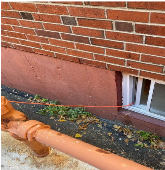
Photograph 8 (left): Unsafe extension cord leaving basement window. Photograph 9 (right): Unsafe extension cord across outside exit ramp.
