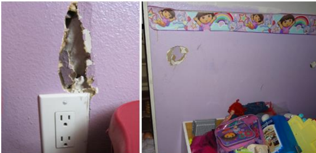
Photograph 4: Holes in the walls of a children's bedroom that a child could reach into.
