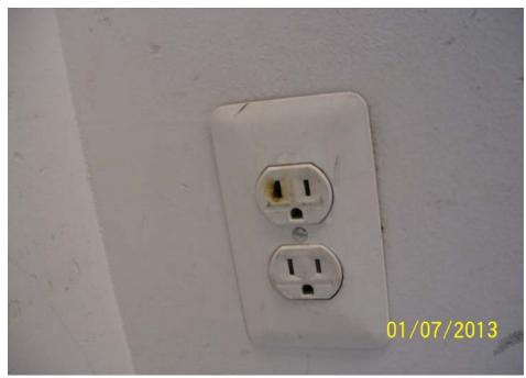
Photograph 2: No protective covering on an electrical outlet.
